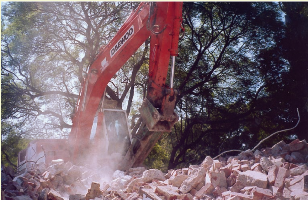
One of the areas of potential risk to silica dust is in the Construction Industry where activities such as sandblasting, tunneling, rockdrilling, jack-hammering and powertool grinding of surfaces containing silica take place.
